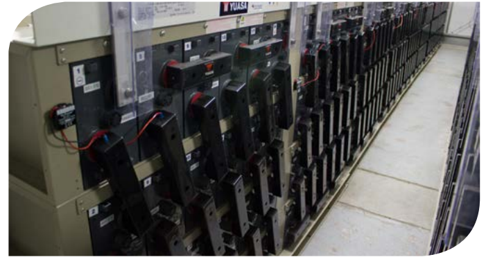
Figure 3.3 Shetland 1MW battery installation
