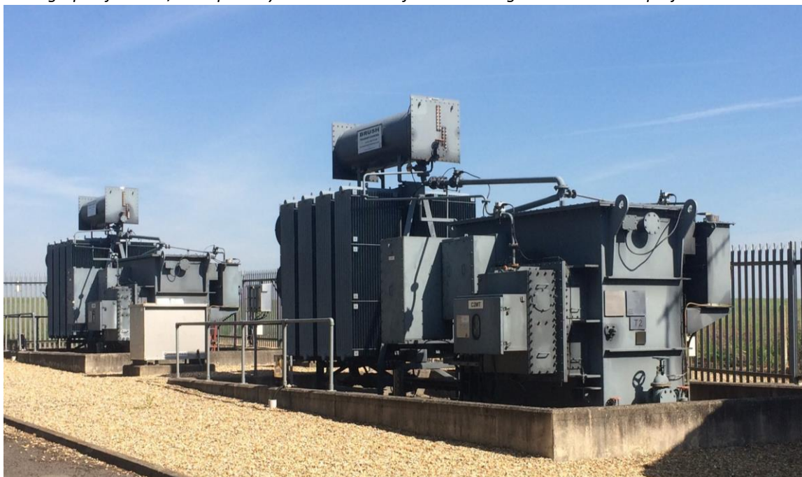
Photograph of two 33/11kV primary substation transformers during a visit to a LEAN project trial site
