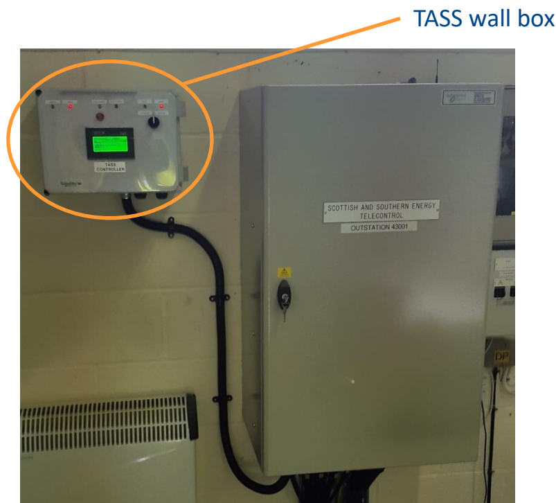
Figure 16 - TASS wall box connected to the RTU within the telecontrol cabinet
