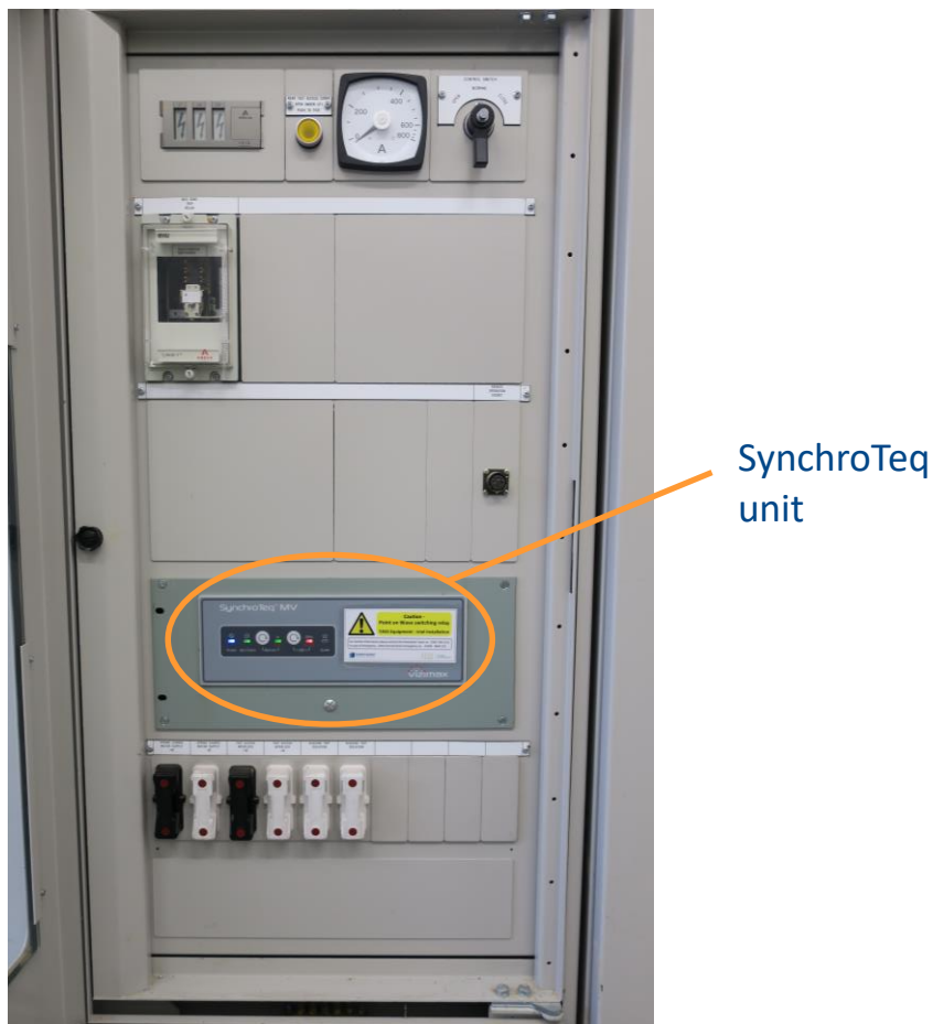
Figure 17 - SynchroTeq MVX relay installed within the switchgear panel
