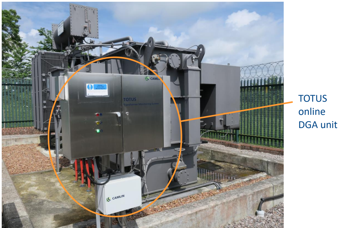
Figure 5 - Online DGA unit installed at a TASS trial site
